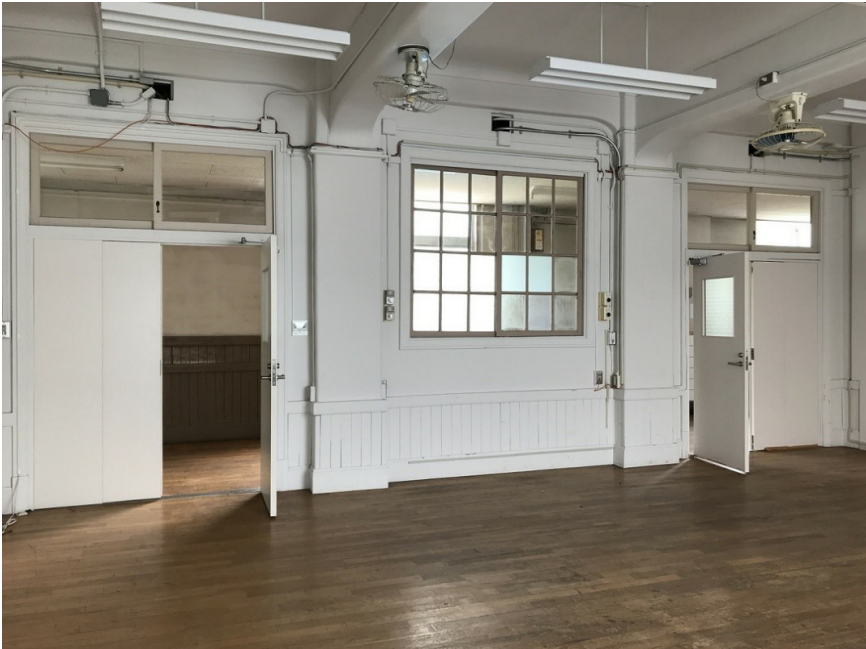
01-01-2F西棟普通教室 廊下側
