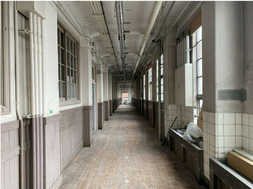
04-01-3F北棟廊下天井
